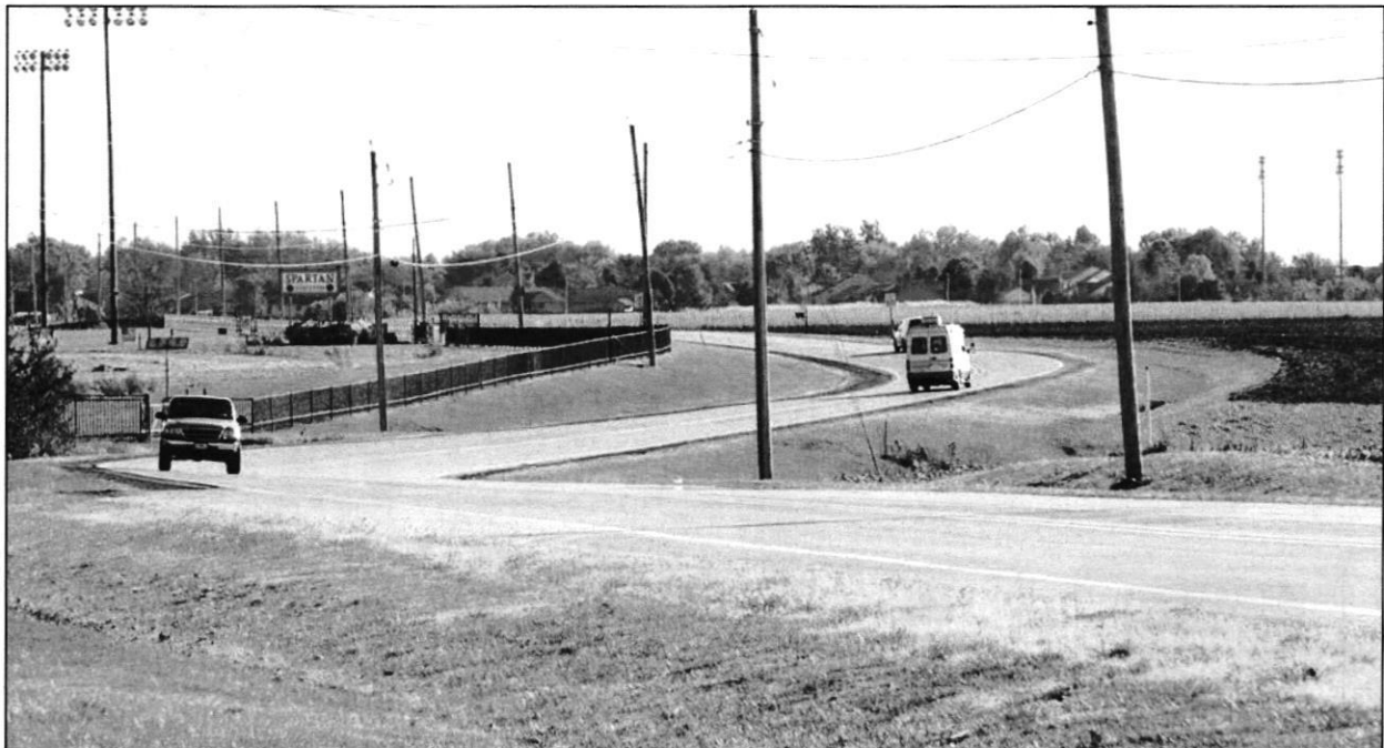
Iron Bridge Road.
